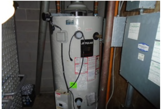
Hot water heater serving the bathhouse was replaced in 2015.
