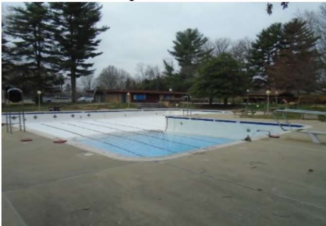
The club has two swimming pools. The wading pool (right photo) is 925 square feet and the main pool (left photo) contains 6930 square feet. The last major pool renovation was in 1996. Both pools were white coated with coping tile repairs in 2019 and are on a 10 year cycle. The condition of the pool piping is unknown. If the piping needs to be replaced, it would require replacement of pool deck.
