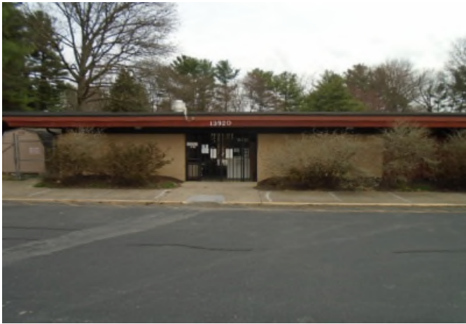
Bel Pre Recreational Association is a private membership club located in Silver Spring, Maryland. Photograph is front view of the building that houses the bathrooms, lifeguard room, and snack bar.
