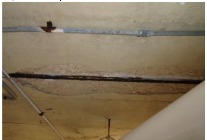
Main pool pump room is located below main pool deck. Roof slab and bearing wall of pump room has possible structural deterioration, and was evaluated by a structural engineer in 2016, who recommended repair of slab and wall damage. Pump room should be repaired or re-evaluated by a structural engineer in the near term. Reserves budget for repairs to be completed in FY23.
