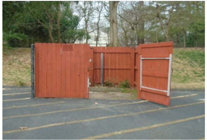
Wood fencing can have its life extended by replacing missing slats, straightening posts and screw fastening loose members.
