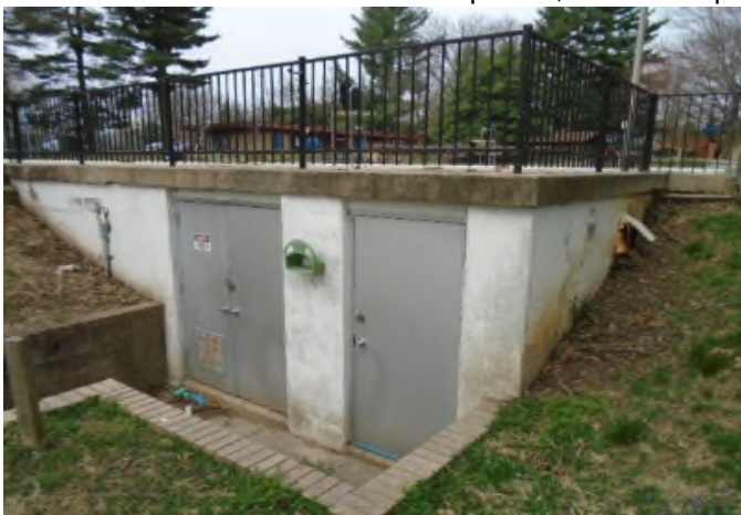
Main pool pump room is located below main pool deck. Roof slab and bearing wall of pump room has possible structural deterioration, and was evaluated by a structural engineer in 2016, who recommended repair of slab and wall damage. Pump room should be repaired or re-evaluated by a structural engineer in the near term. Reserves budget for repairs to be completed in FY23.
