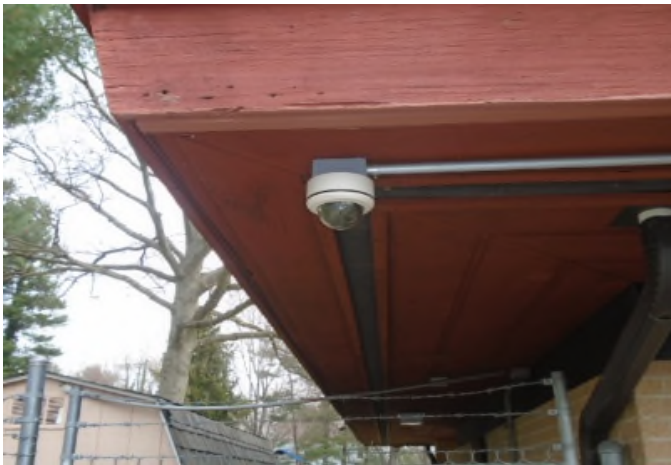
Security system is included in the reserves. Repair/replacement will be needed when parts are no longer available or system reliability is compromised.
