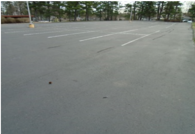
Pavement is holding up well. Parking lot was last milled/overlayed in 2008. Crack filling most recently done in 2020. See our recommendations in the comments section for proper care of asphalt pavements.
